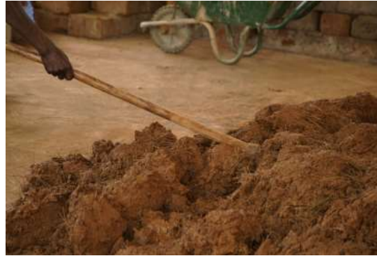
Figure 11. Mixing of mud with fibres
