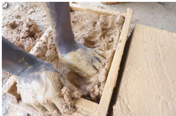
a) Compacting mud into mould in 3 layers
